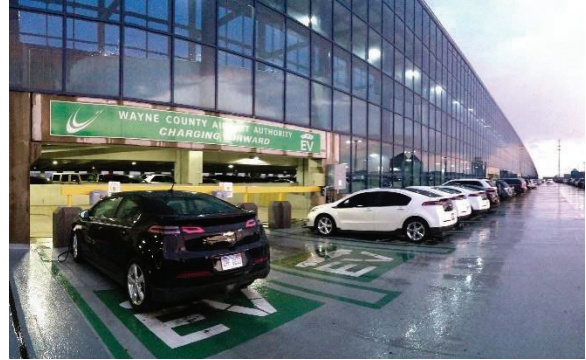
Photo: Electric Vehicle (EV) Charge Ports at the Blue Deck
