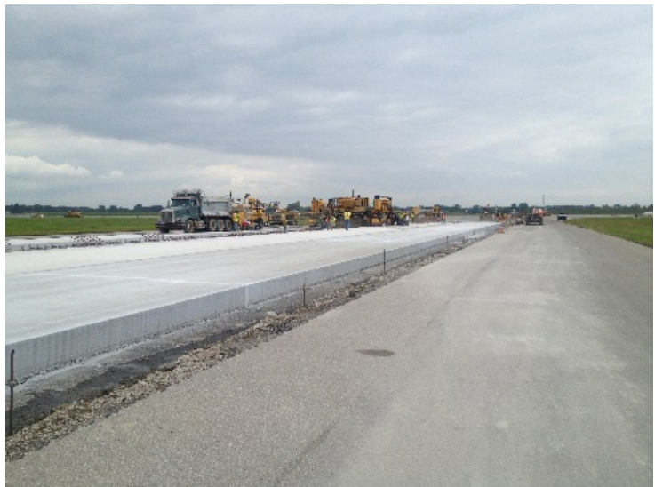
Picture H - 1: Taxiway V
