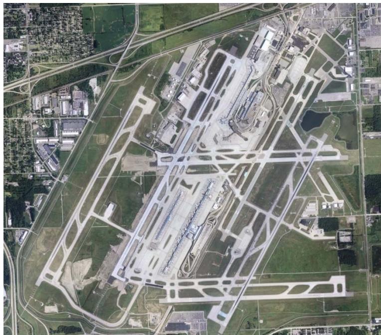
Photo: Aerial Photograph of the Airport, August 2013
