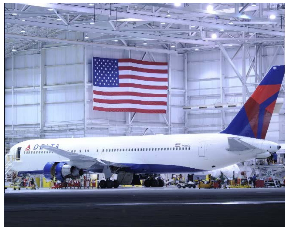
Photo: Delta Hangar
