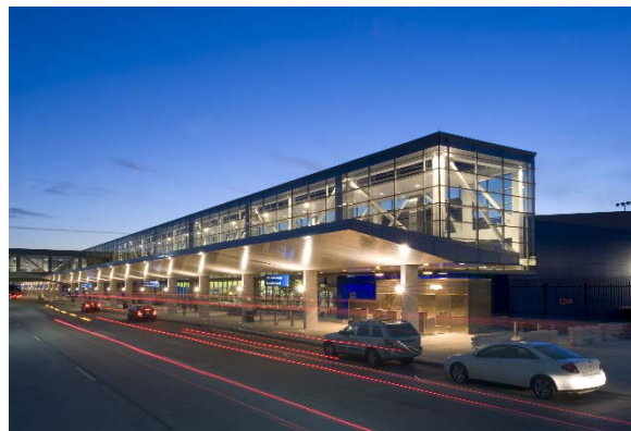
Photo: North Terminal
