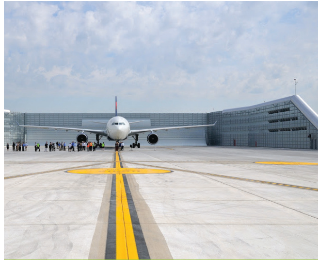
The DTW Ground Run-Up Enclosure (GRE).
