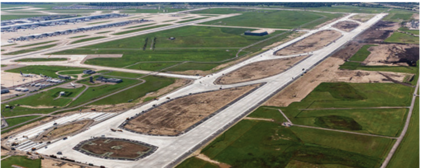
Aerial view of Runway 4L/22R Rehabilitation Project.
